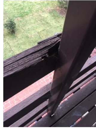
Rotting handrail/balustrade
