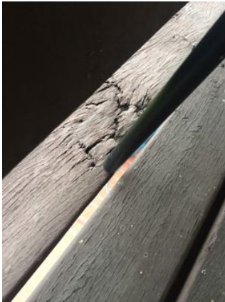
Rotting deckingboards
